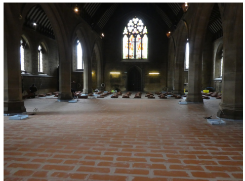
St Andrew's, Kettering, with the new floor substrate in place
