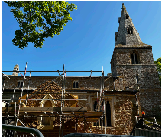
Exterior of All Saints', Wilbarston, during work on the new access
