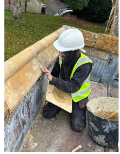
Work underway at Moulton
